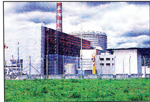
Fig. 3.16 : Nuclear power station, Kalpakkam
