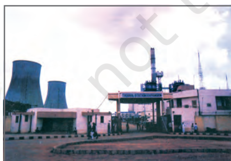
Fig 3.10: A view of a Thermal Power Station
